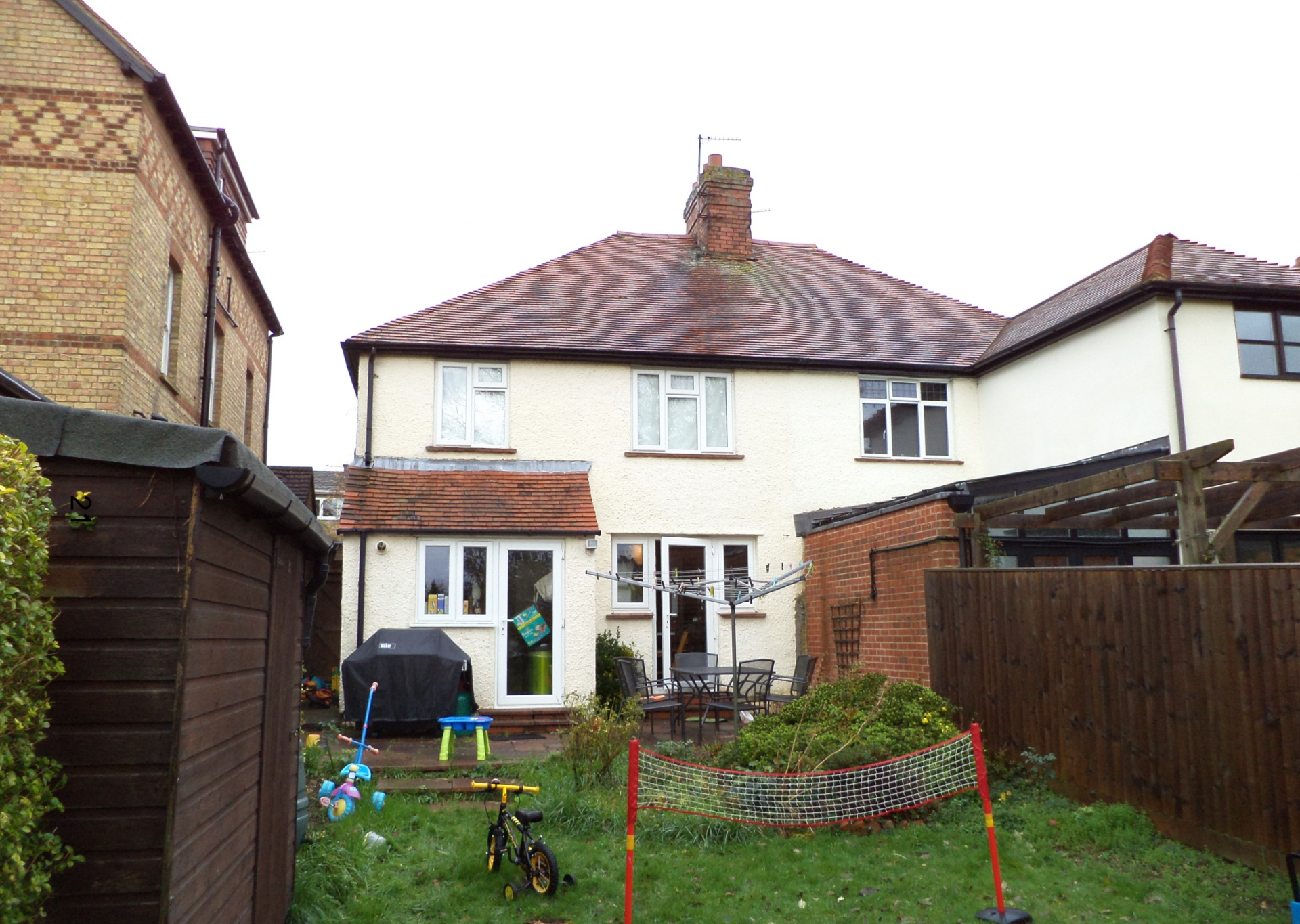
View of rear of property
