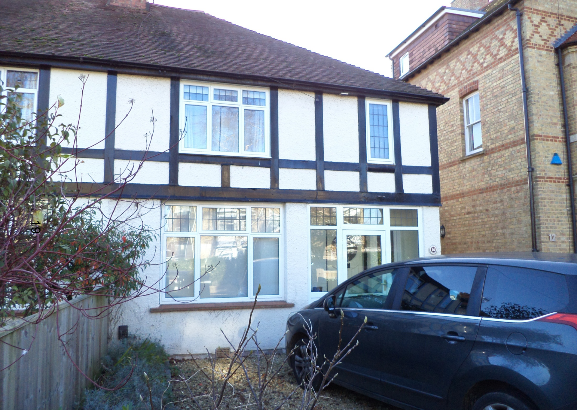
View of front of property
