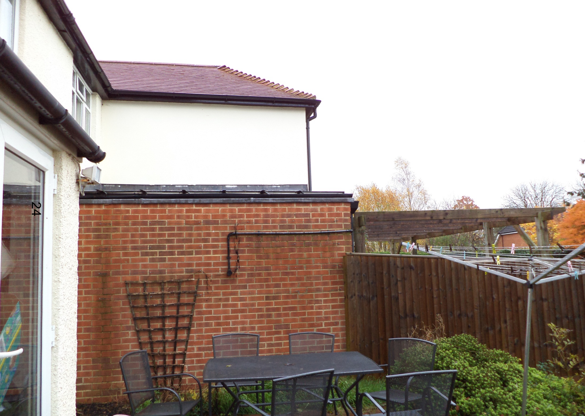
View from property to rear extension at 16 Hernes Road
